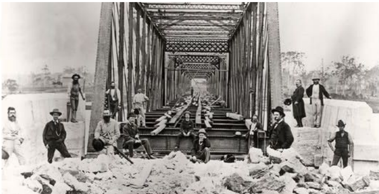
Building The Bridge II
