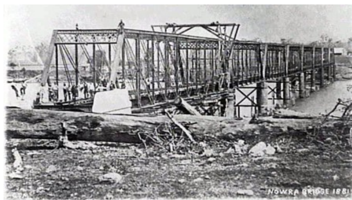
Building The Bridge I
