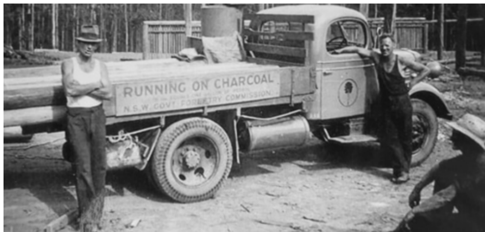
A gas producer on a NSW Forestry Commission truck
