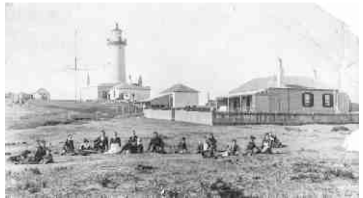
Cape St George Lighthouse, originally on the southern peninsula of Jervis Bay
